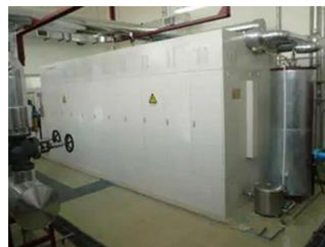
Electric heat storage boiler
